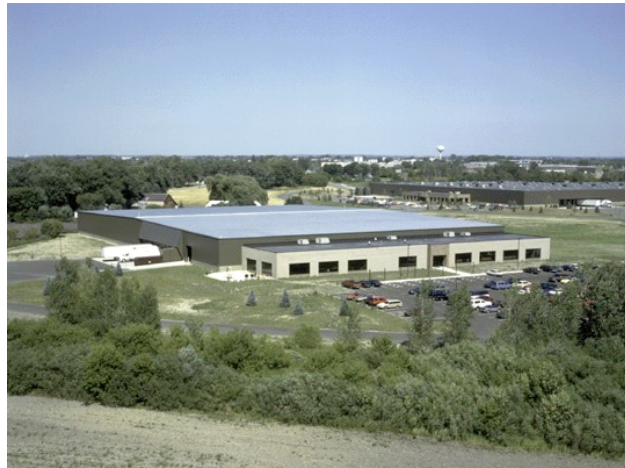
Johnson Controls Li-ion Cell Manufacturing and Battery System Assembly Plant, Holland, Michigan
